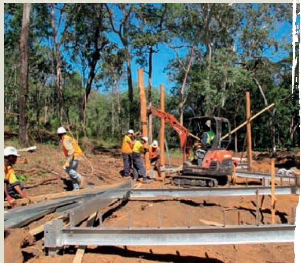
The Shipton’s Flat ranger base from the ground up.
